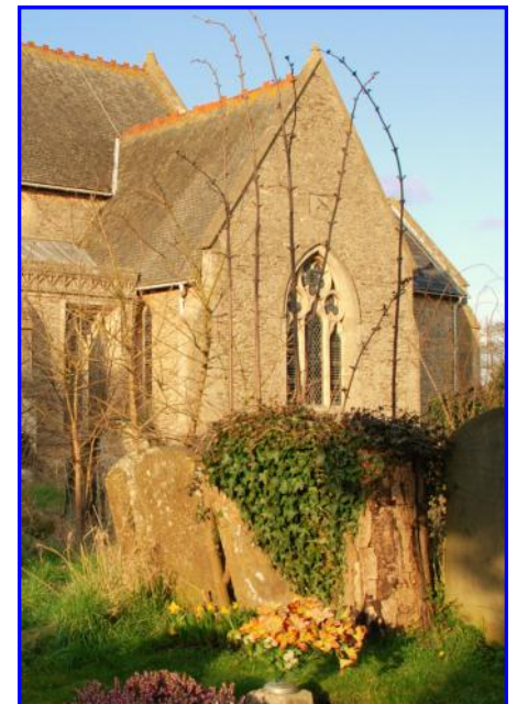
St James Church, south elevation in winter sun
