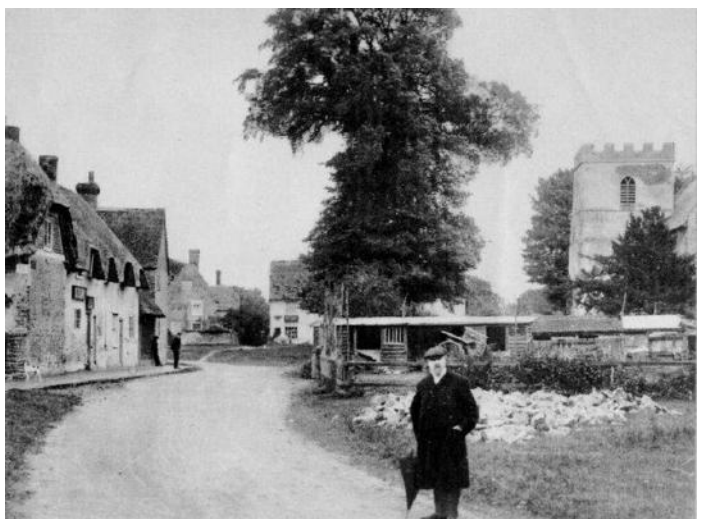
Church St, West Hanney, looking east.
